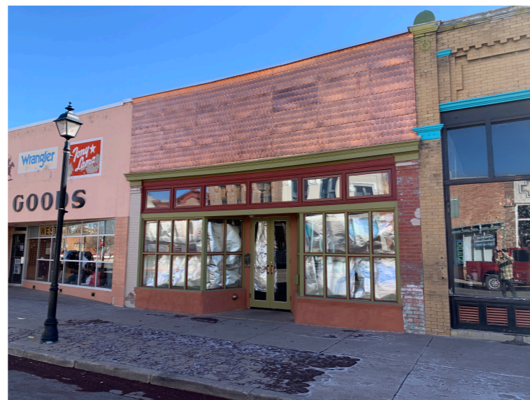
Rehab Underway, Bridge Street
