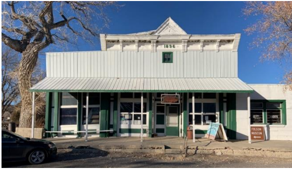
Village of Folsom's Restoration of Historic Doherty Mercantile Building and Folsom Museum - 2021
