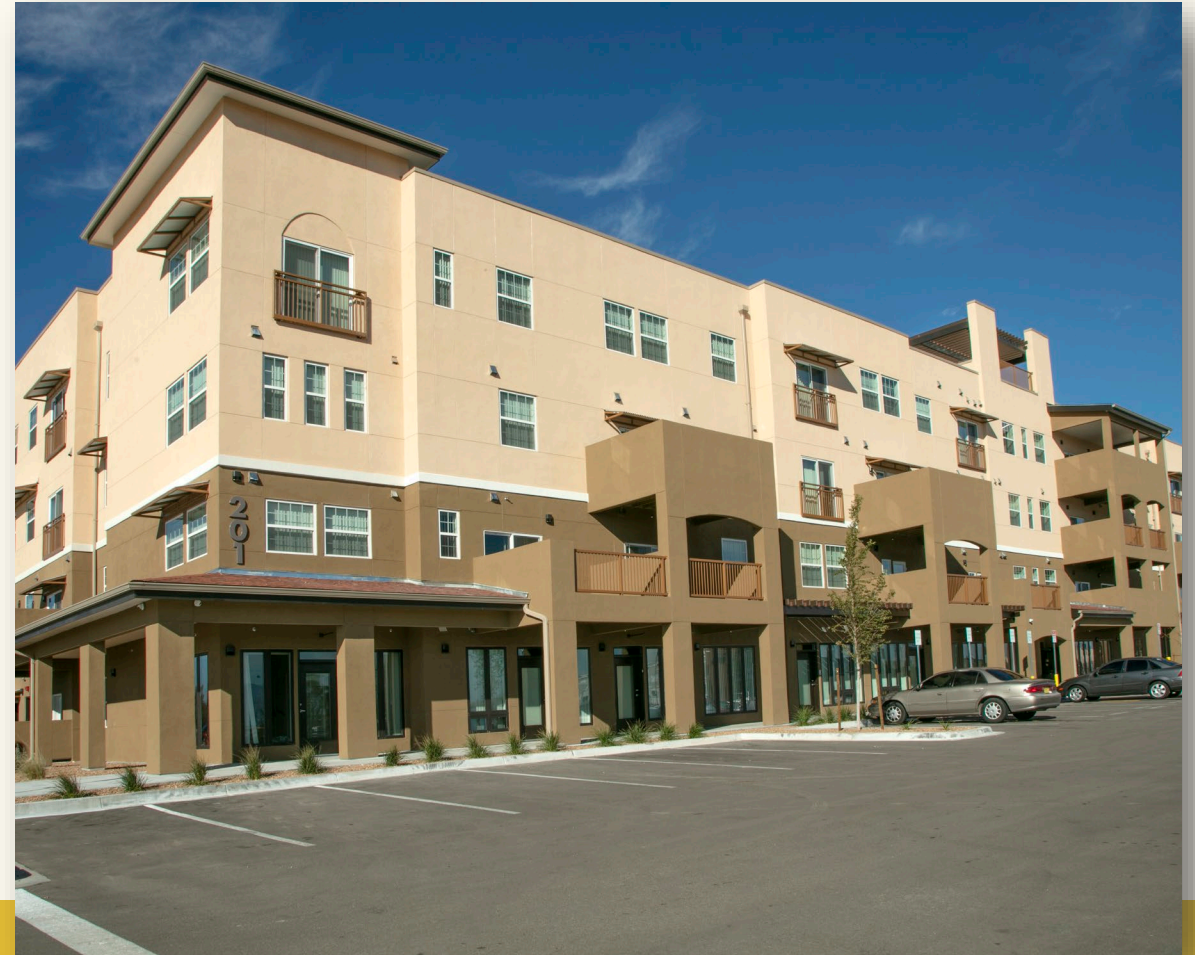
Residential construction completed September 2020.
