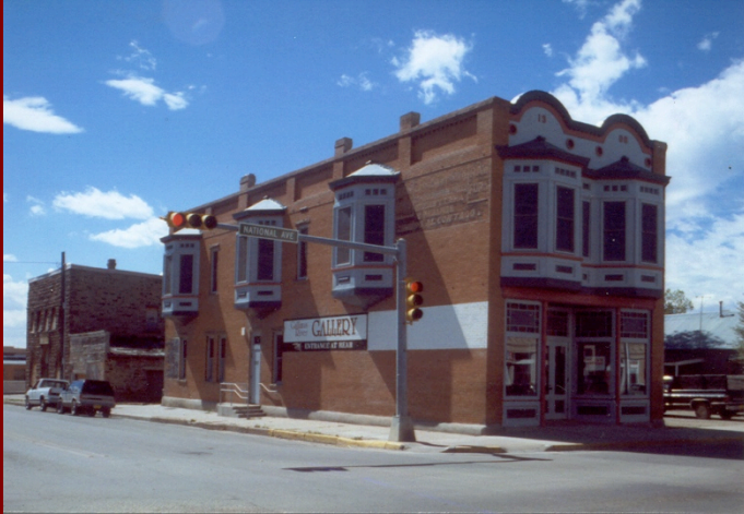
TAICHERT BUILDING LAS VEGAS, NM
