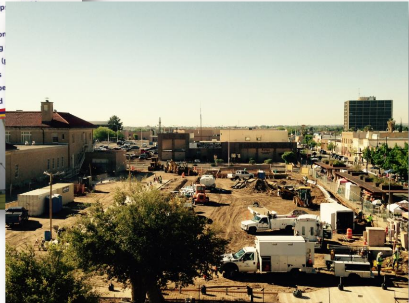
Downtown Las Cruces Plaza Under Construction, April 2016
