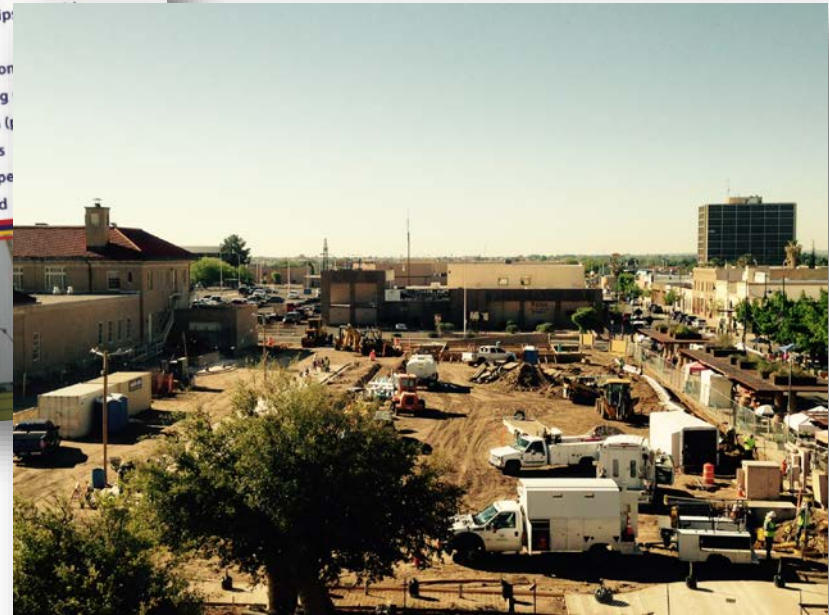
Downtown Las Cruces Plaza Under Construction, April 2016
