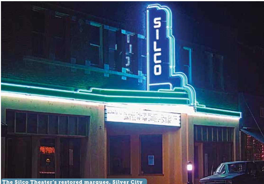
The Silco Theater's restored marquee, Silver City
