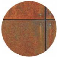
Weathered Steel Wall
