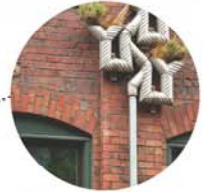
Artful Roof Drains for Irrigation
