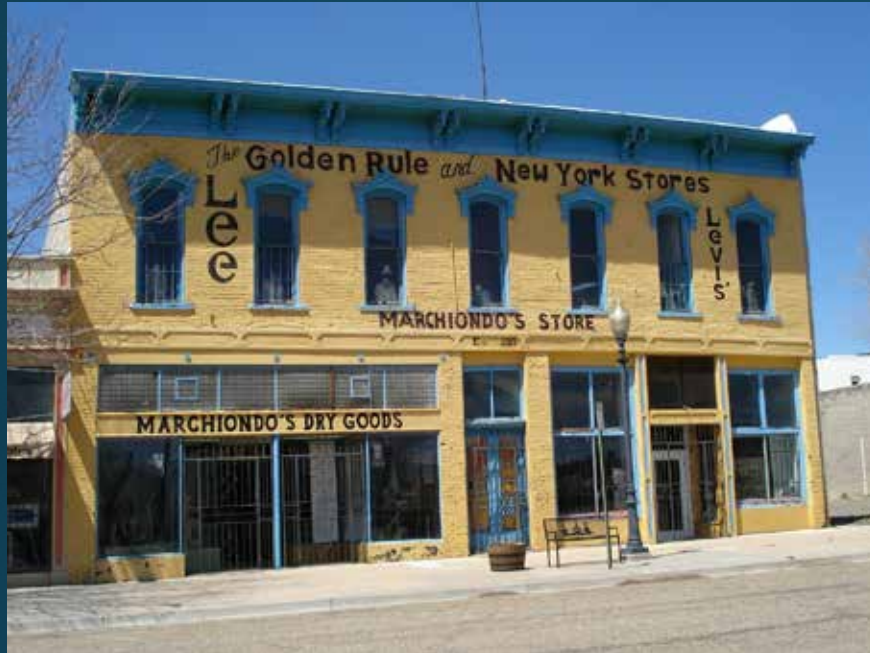
Marchiondo Building Retail + Studio Lofts
